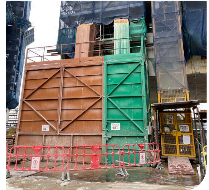
The bespoke double refuse chute that facilitated better sorting
