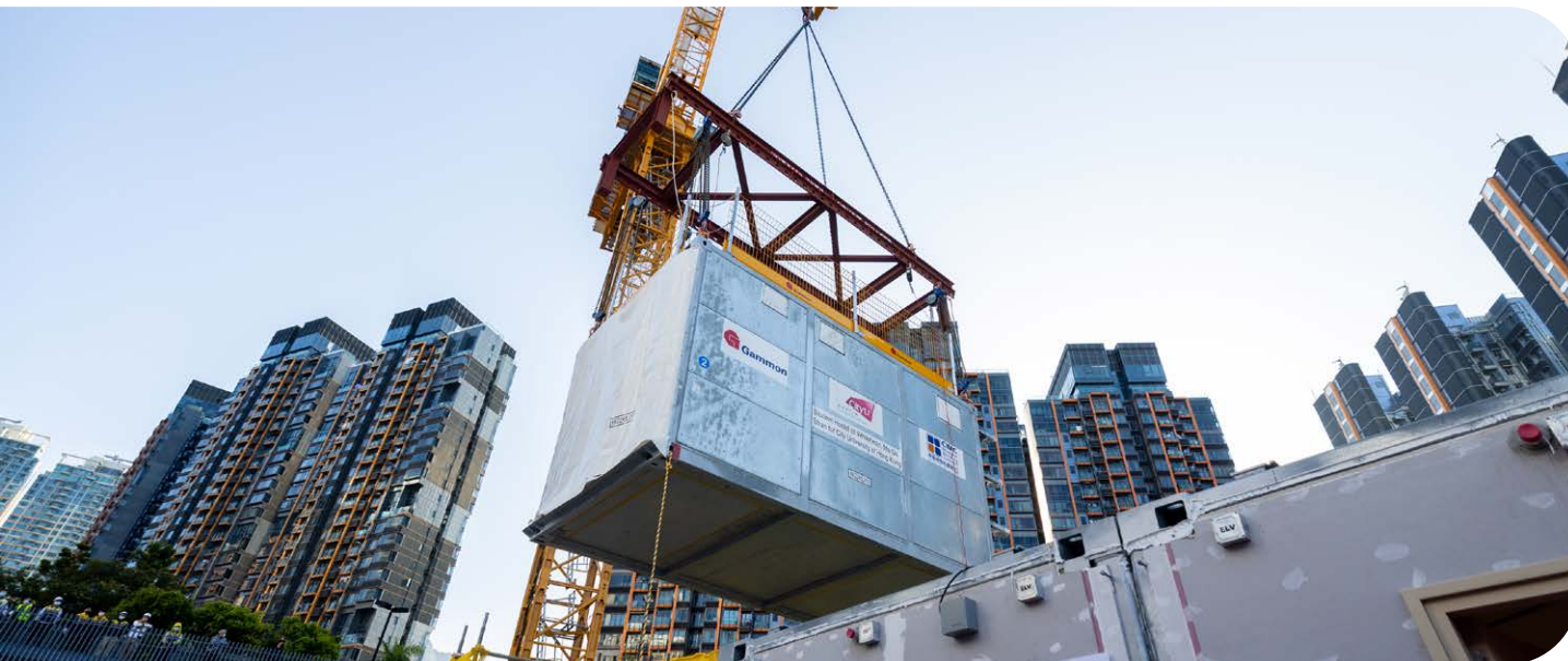
An MiC unit is lifted into position on our CityU student hostel project
